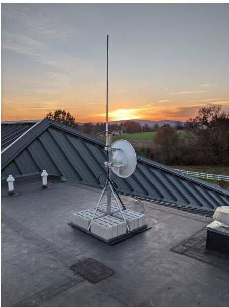
One of the CCAR microwave nodes located
